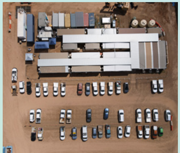
Construction compound for big battery site
